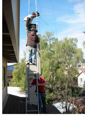
Doug and two professional roofers work together to re-install the antenna.
